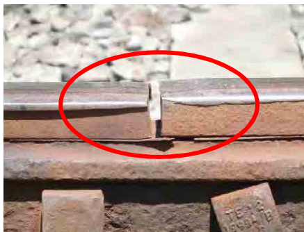
Figure 3.1.6 Deformation of Rail
