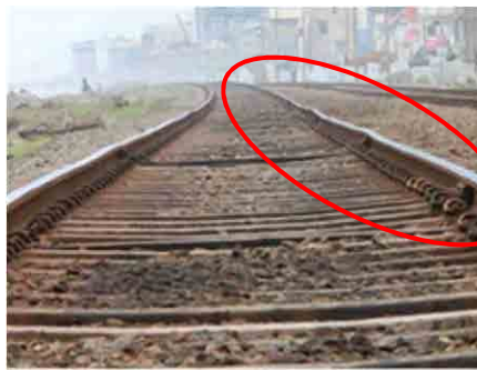
Figure 3.1.7 Irregularity of Alignment
