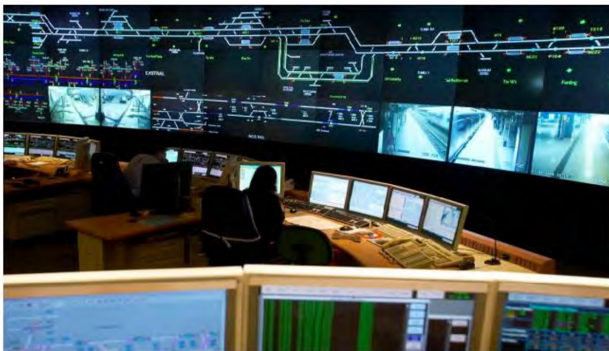
Figure 11-6 OCC Showing Video Wall Overview Display (IRSE, 2010)
