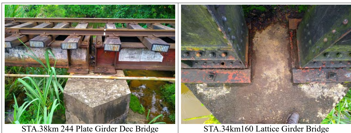
Figure 8-7 Bearings of Existing Bridge Structures
