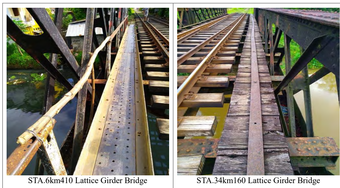
Figure 8-10 Handrails and Walkways of Existing Bridges
