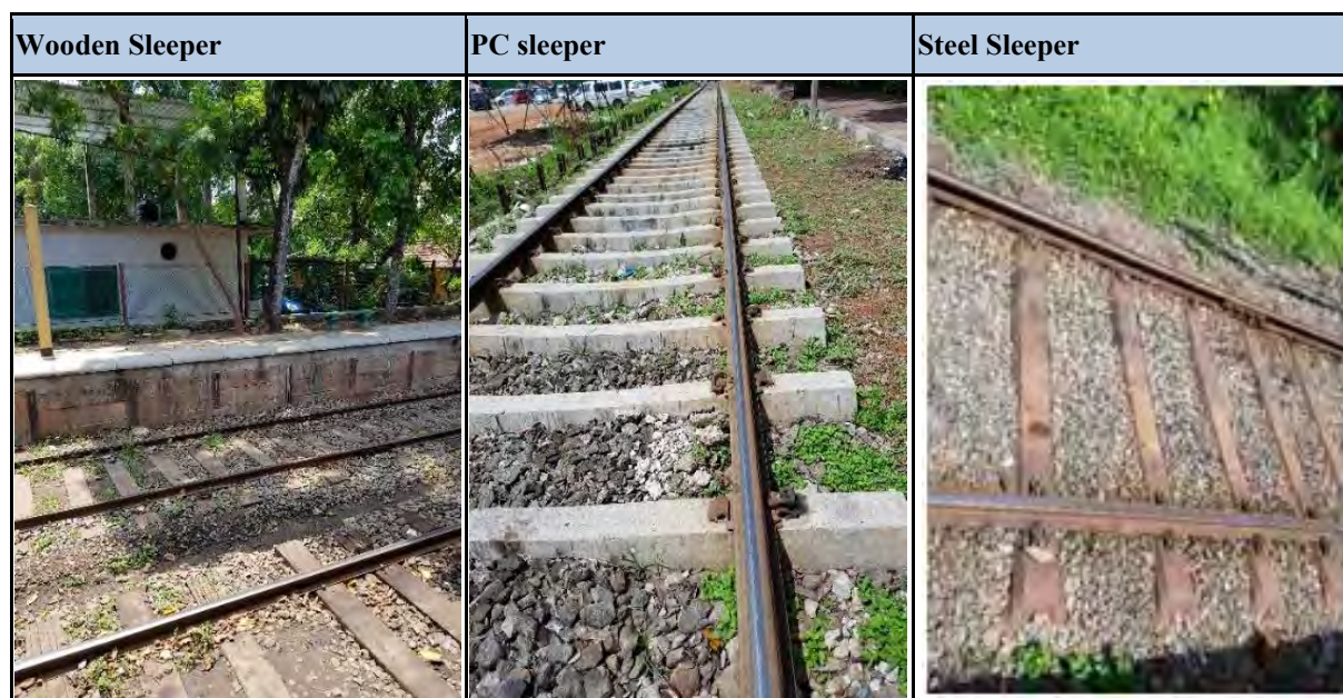
Figure 9-1 Track Condition in Main line and Stations
