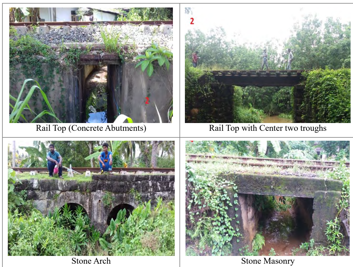
Figure 8-5 Existing Culvert Structures of Kelani Valley Line
