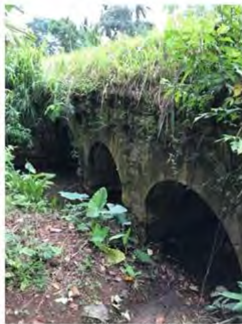
Typical Arch Rail Culvert
