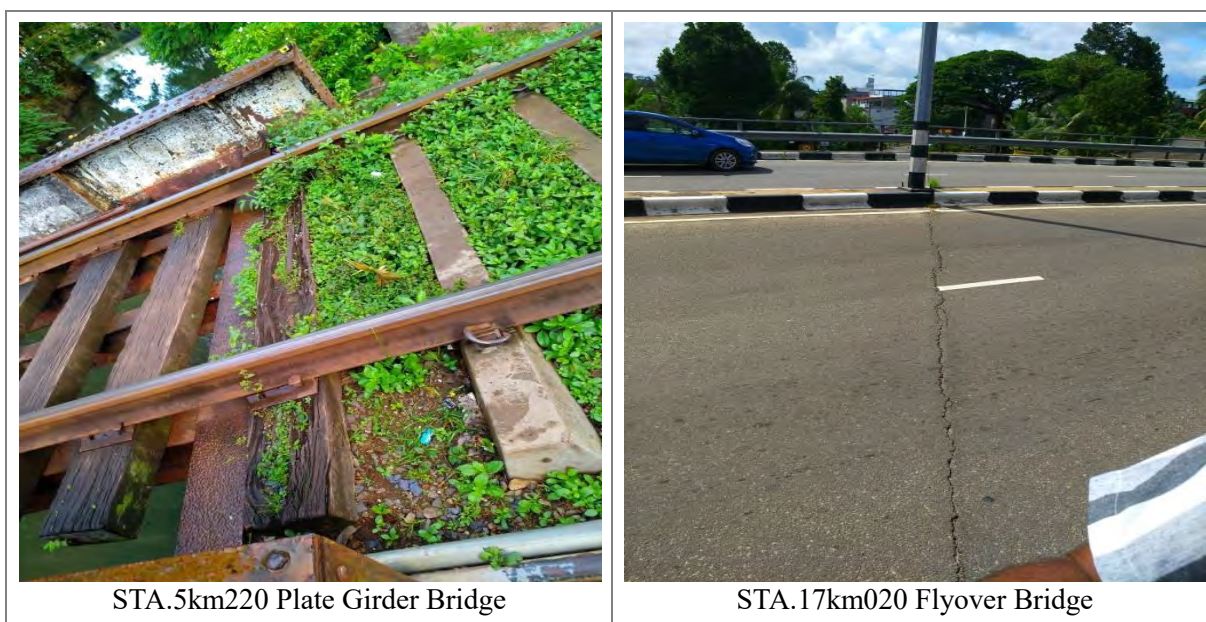
Figure 8-8 Expansion Joint of Existing Bridge Structures
