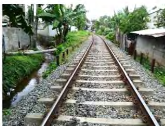
A Drain Parallel to the Railway
