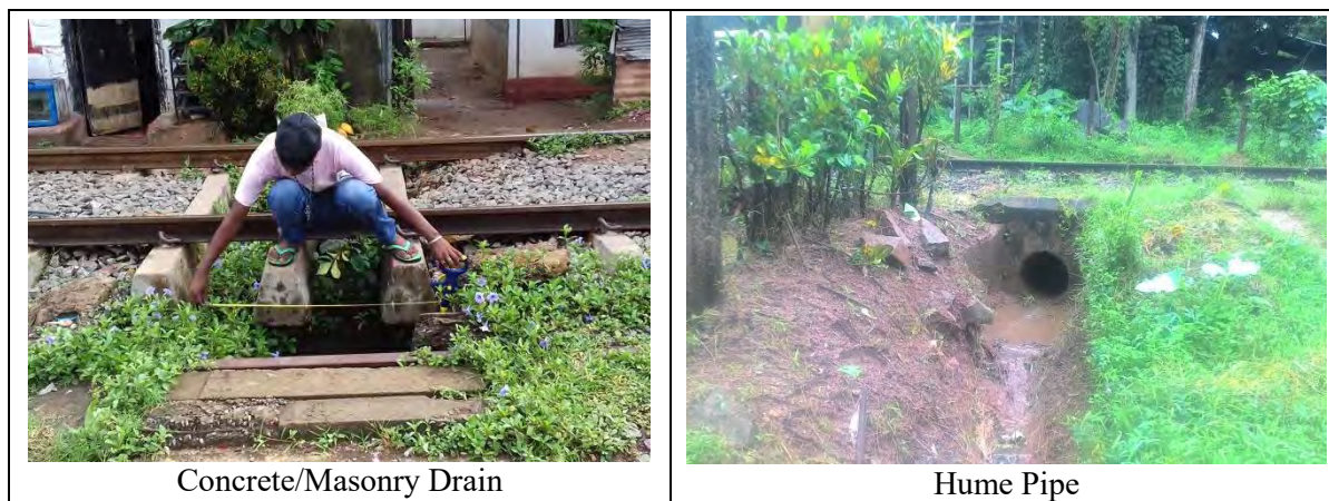
Figure 8-6 Open Drain across the Railway Line
