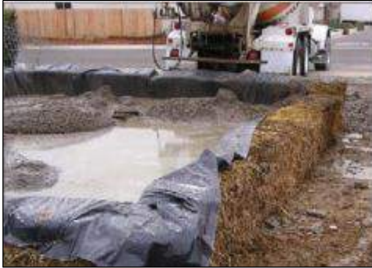
Figure 24: A Sample of a Concrete Mixer Truck Wash Water and Sludge Drying Bed (source: www3.epa.gov/npdes/pubs/concretewashout.pdf )
