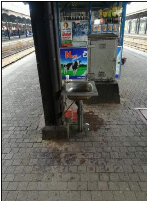
Figure 4: Improperly Built Drinking Water Fountain and Platform Deck (Colombo Fort and Maradana Stations)
