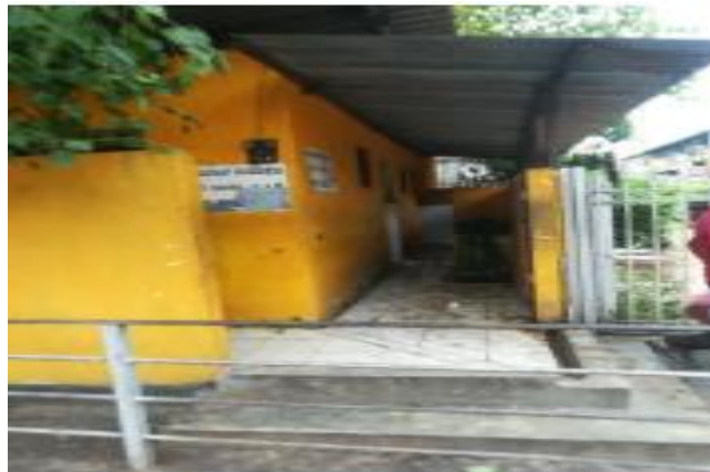
Figure 1: An Existing Toilet Facility at Colombo Fort Railway Station (With Poor Sanitary Conditions)
